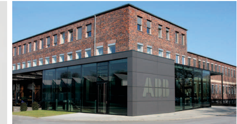
The Stotz Kontakt factory (Heidelberg, Germany)
